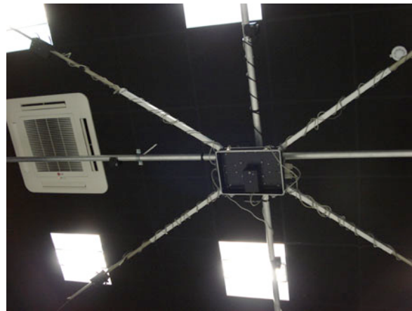
Fig 2. The 5 Cricket receivers on their extendable grid in the ceiling
